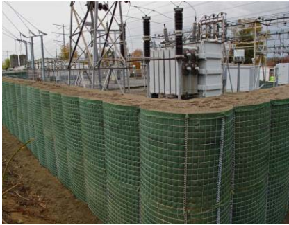
Flood Barrier Source: Con Edison
